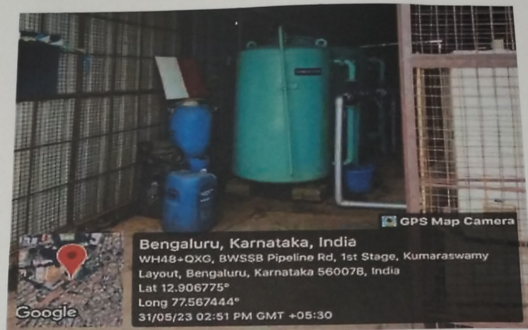
SEWAGE TREATMENT PLANT
